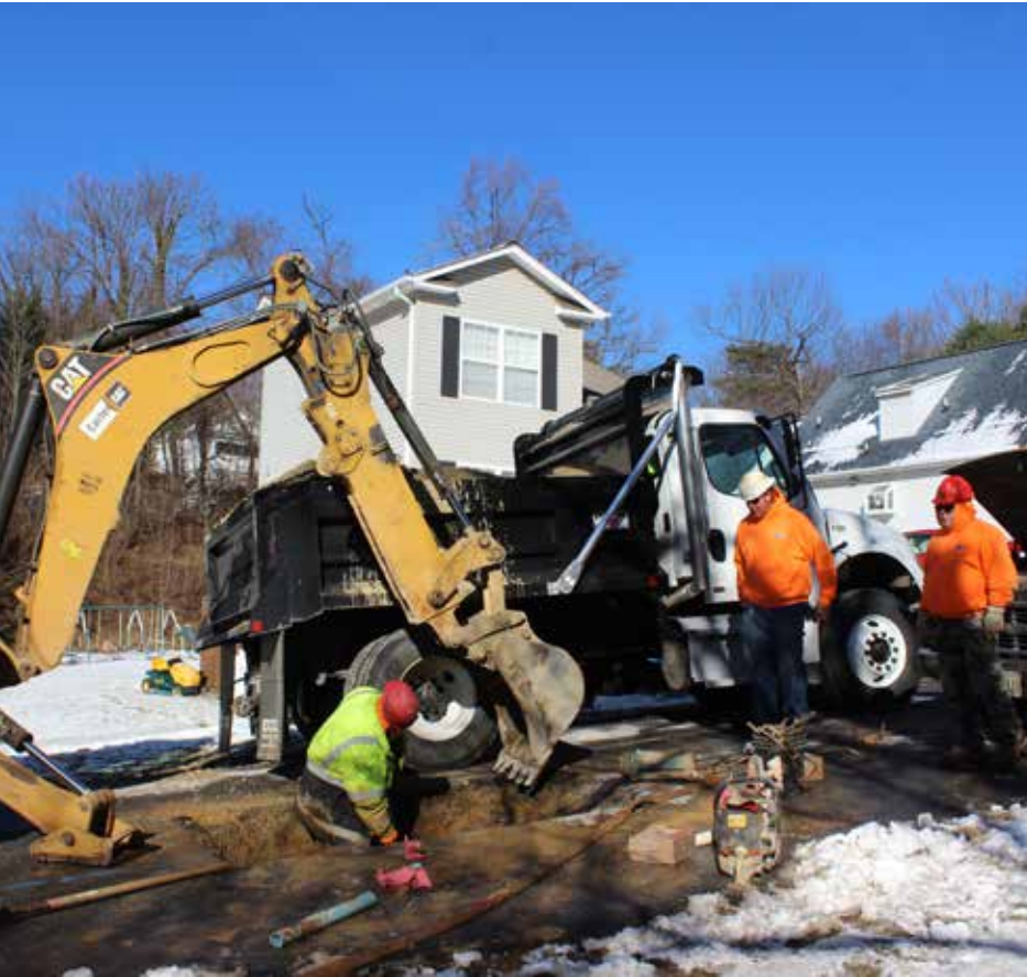
The Water Department worked quickly to repair main breaks, like this one on North Stonewall Street, that were common during the winter months.
